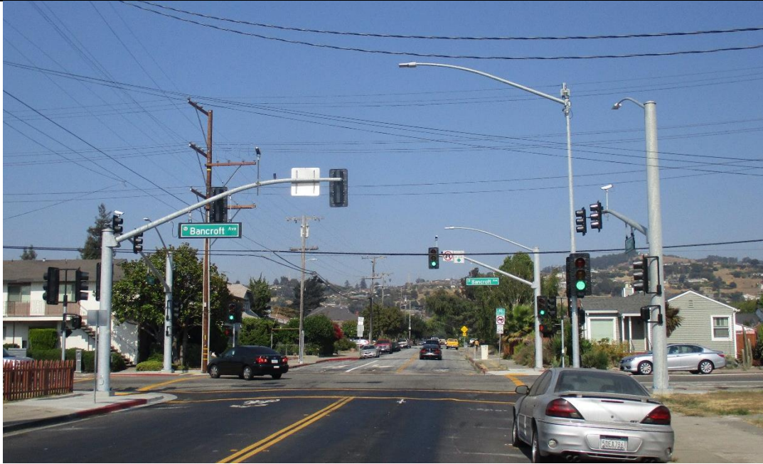
NEW SIGNALS, BANCROFT – SYBIL INTERSECTION
